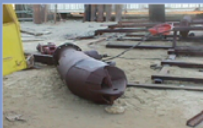
Pipeline pulling head
