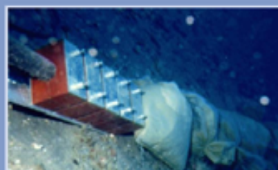
Anchor system and sand bagging
