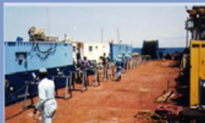
Rig-up of cable, drum & Rollers
