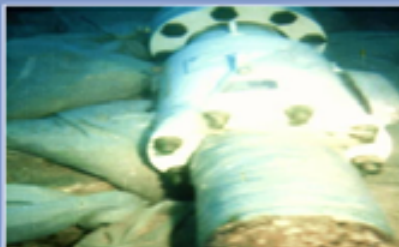
Supporting of repaired pipeline
