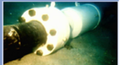
Repaired pipeline by a mechanical connector
