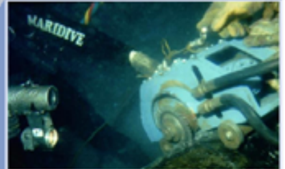
U/W pipeline cutting
