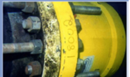
Bolt Tensioning of connectors
