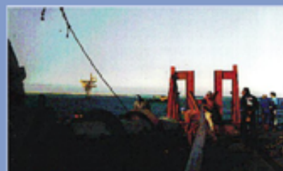
Pipe techener & Rollers
