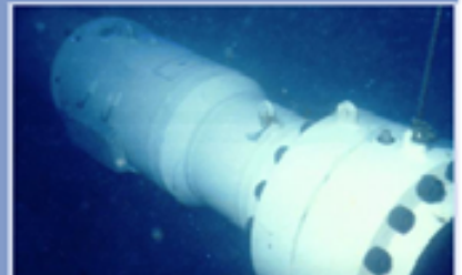
Mechanical connector after installation
