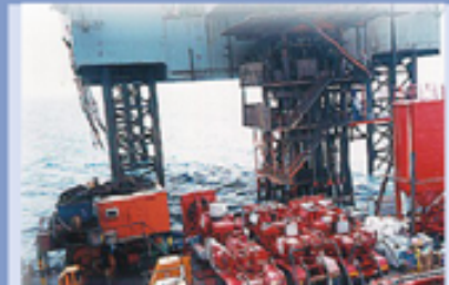
Barge & Rig during Frac job
