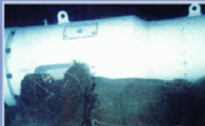
Mechanical connector installation
