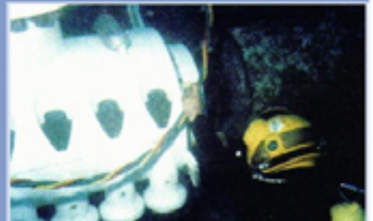
T- clamp installation on pipeline
