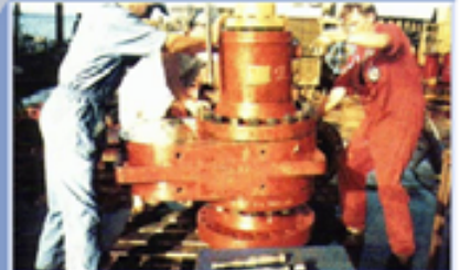
Preparation of hot tapping machine
