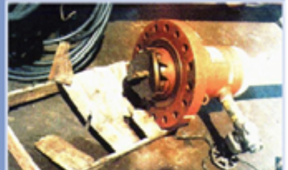
Tapping Machine and cutted pipe coupon
