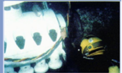
Tightening of the packing flange
