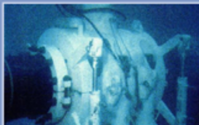
Leak test for T-clamp
