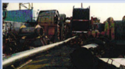
Pipe reel on laying machine
