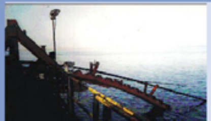
Tube a large Barge Stenger
